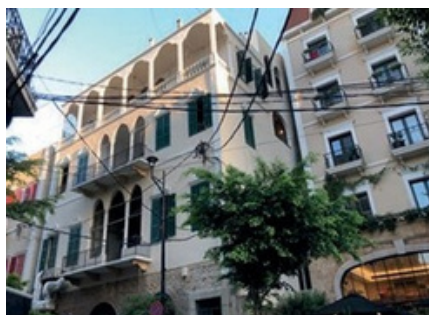
Rmeil 400 North Block
